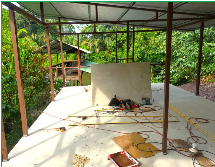
2nd floor - Roof installed with bird's nest of dock in background
