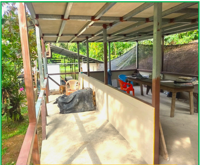
2nd floor - Ceiling installed with dock in background
